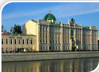
26/1, Sofiyanskaya Embankment, Moscow
